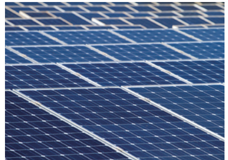
Solar Array Load Testing
